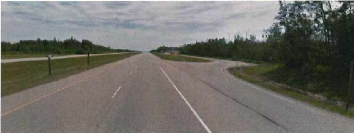
Viewing east in EBL's, west of the intersection. There is an intersection 400m west of the RR 32 intersection that connects to a service road that accesses RR 32.
