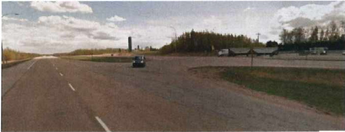
Viewing east from the WBL's, just west of the intersection.
