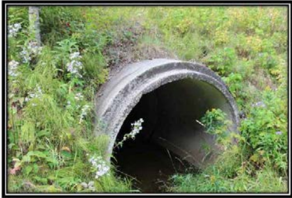
Photo 19: Water in the culvert at the crossing site in the northwest.
