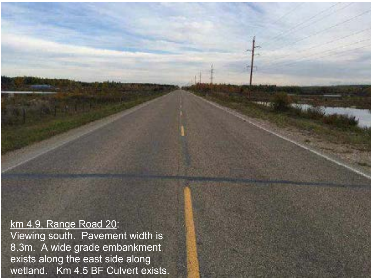
km 3.7, Range Road 20: Viewing south. Pavement width is 8.3m. Lac Ste. Anne County approx. at km 3.6. Brush growth within ROW on west side.
