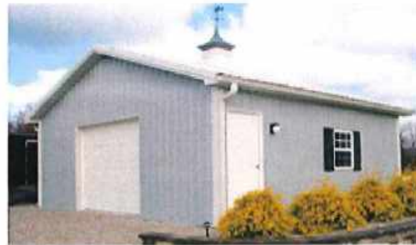
Typical Utility & Maintenance Building
